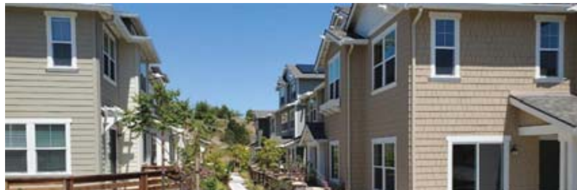
One example of multi-unit housing
