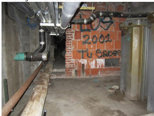
Back end of main tunnel Photo Vera Kochan
