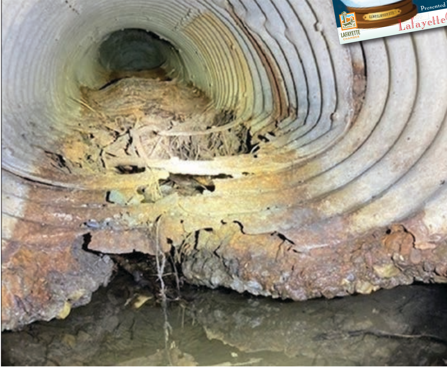
Corrugated metal pipe deterioration of invert near Donald Drive and Moraga Road.
