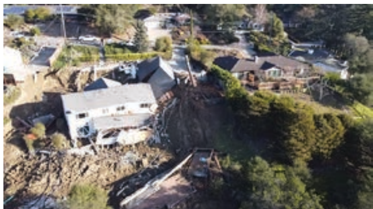
Damaged homes on Cedar Lane in Orinda Photo courtesy city of Orinda
