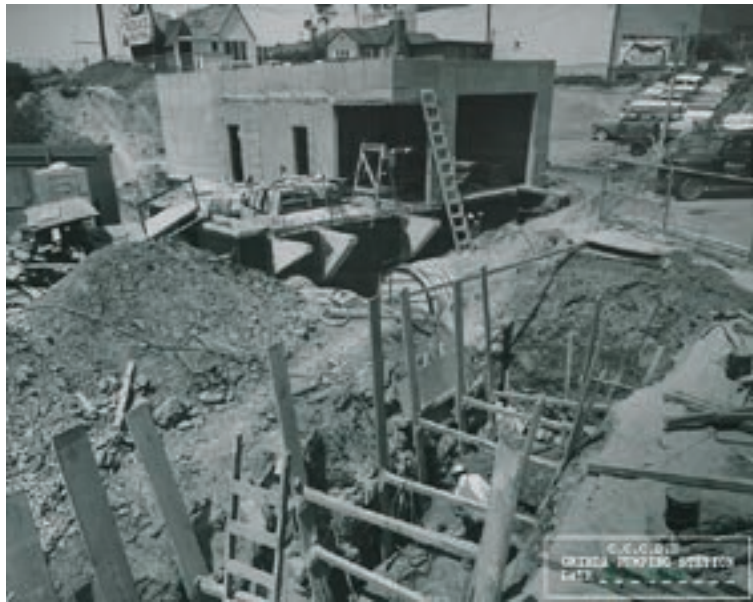
Orinda Pumping Station in 1960
