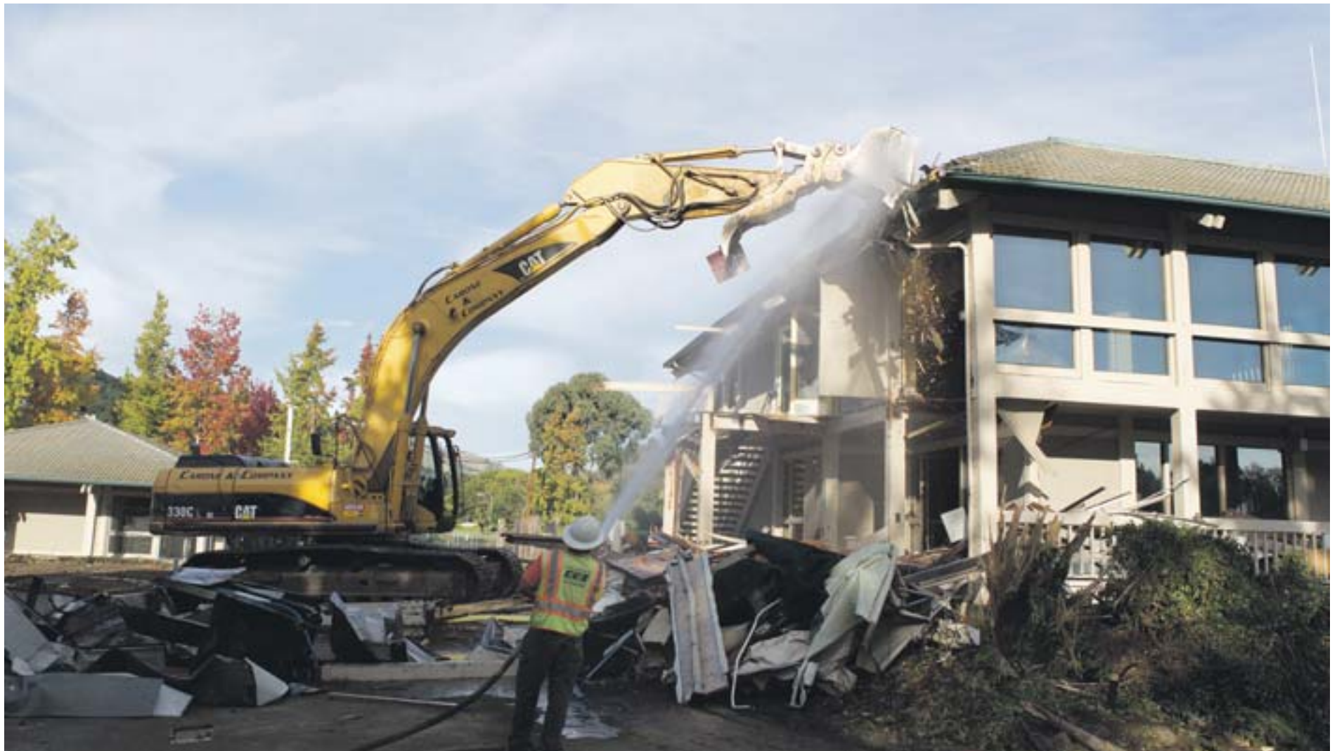
Excavator takes the first bite of the club house roof
