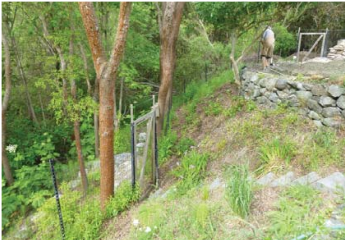
The Sorensons' creek restoration
