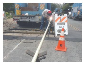
A PG&E welder cuts a new steel lateral for installation. Photo Victor Ryerson
