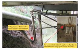
A landslide reached and damaged the Canyon Bridge foundation. Photo provided
