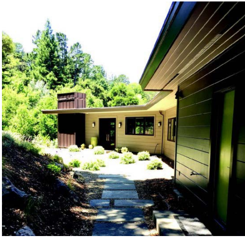
An overhang shades the front entrance of this mid-century modern home. Photo courtesy April Matthews
