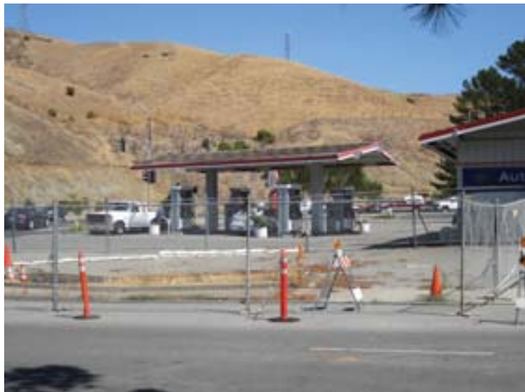
Rheem sinkhole still awaits repairs.
