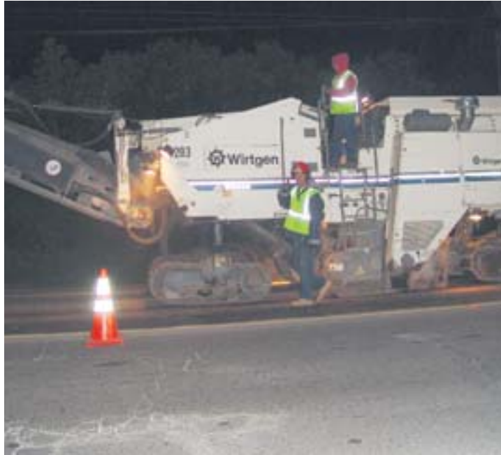
Night work on Moraga Way
