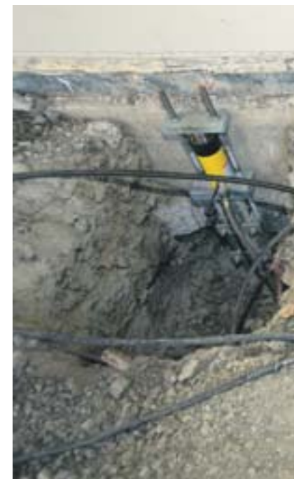
Lift set up
