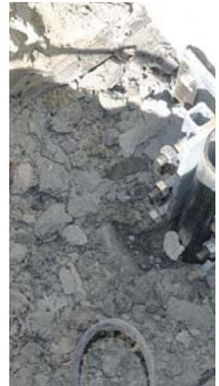
Installed pier pipe
