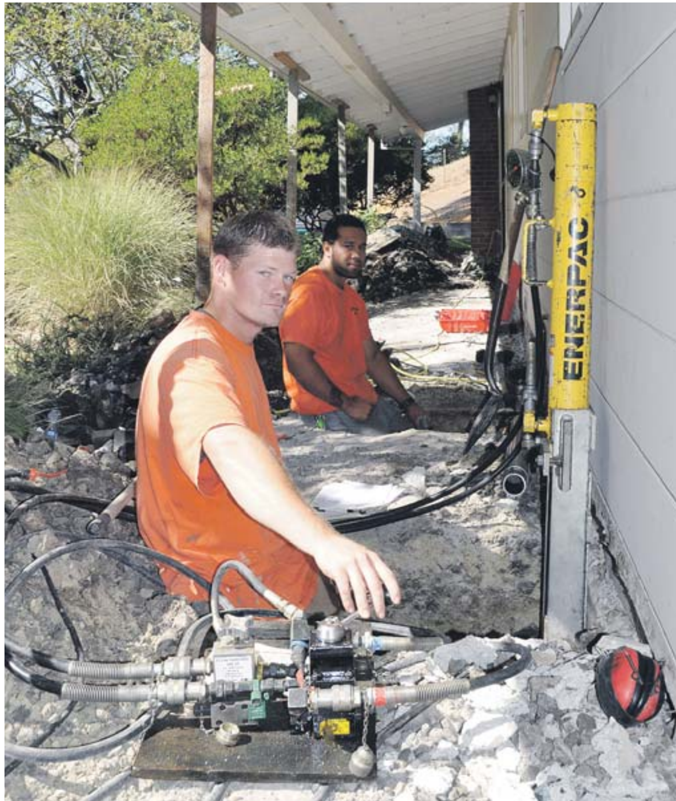
Michael Mahoney and Sergio Navarro doing drive stand & pier installation
