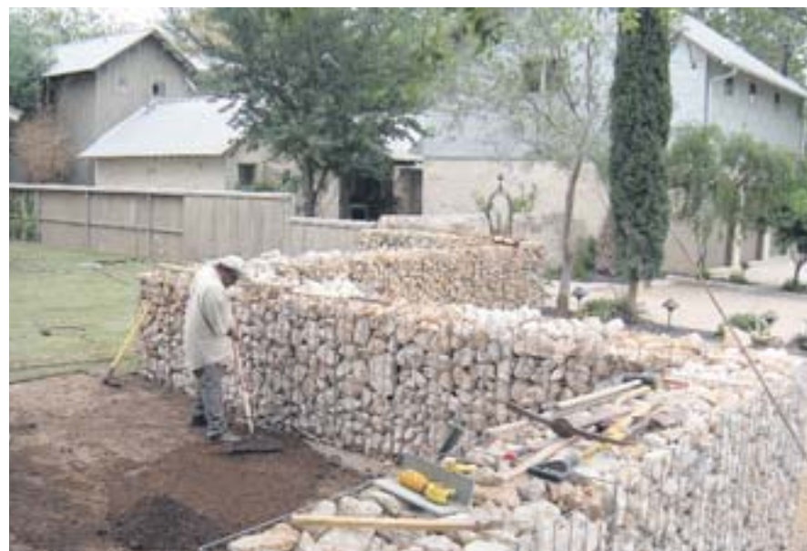
Building a gabion wall
