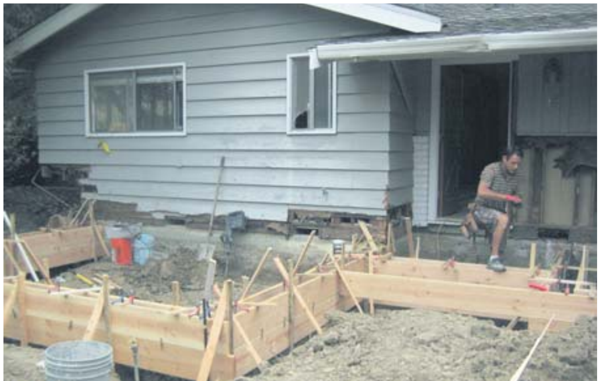
Daniel Leleu builds a new foundation at the front of the home.
