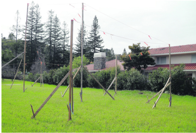
Story poles of proposed home on Las Huertas Road. Photo C. Tyson
