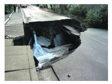
Last weekend's heavy rains, a leaky water pipe and a clogged culvert that caused water to pool on Mountain View Drive eroded and undermined the roadway creating a large sinkhole that may take months to repair permanently.
