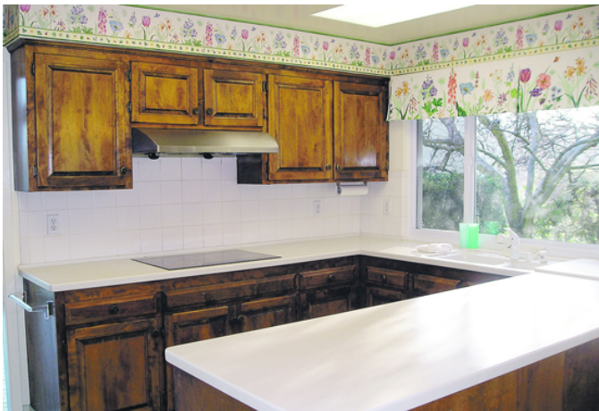
"Before" shot of a 1970s era fused acrylic solid surface counter. Photos Cathy Dausman
