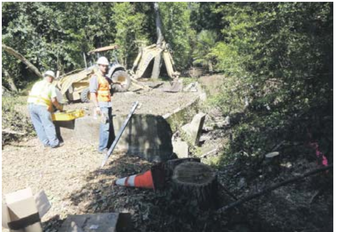
Michael Vidra from BKF supervises the removal of concrete blocks from Laguna Creek. Photo Sophie Braccini
