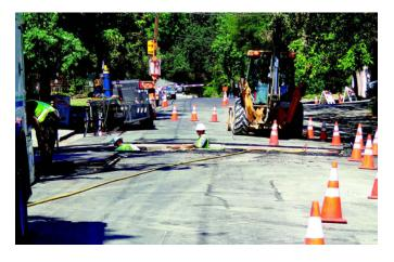
Brook Street is closed near Moraga Road for EBMUD, where workers are replacing over 500 feet of pipe that was installed in 1933. Photo Cathy Tyson
