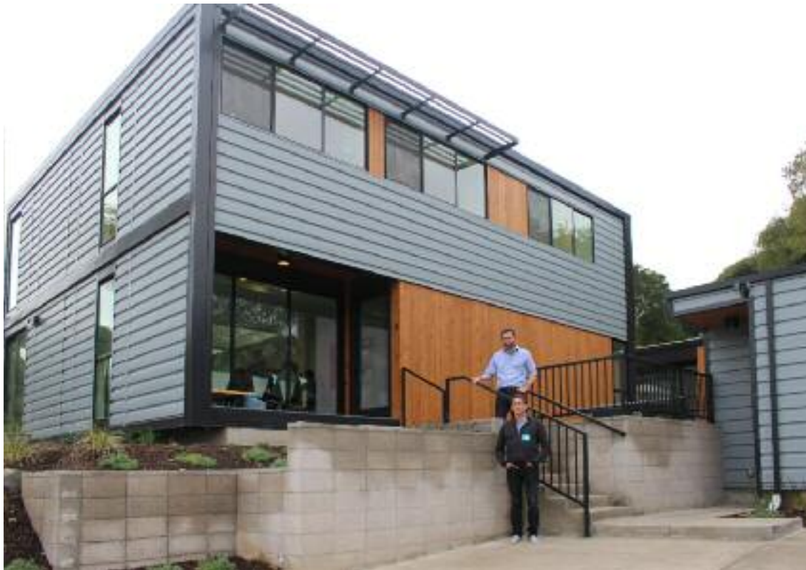
Jared Levy, below, and Gordon Stott, above, of Connect-Homes in front of a modular home in Orinda that was built customized for the family then constructed on site. Photo Chris Lavin
