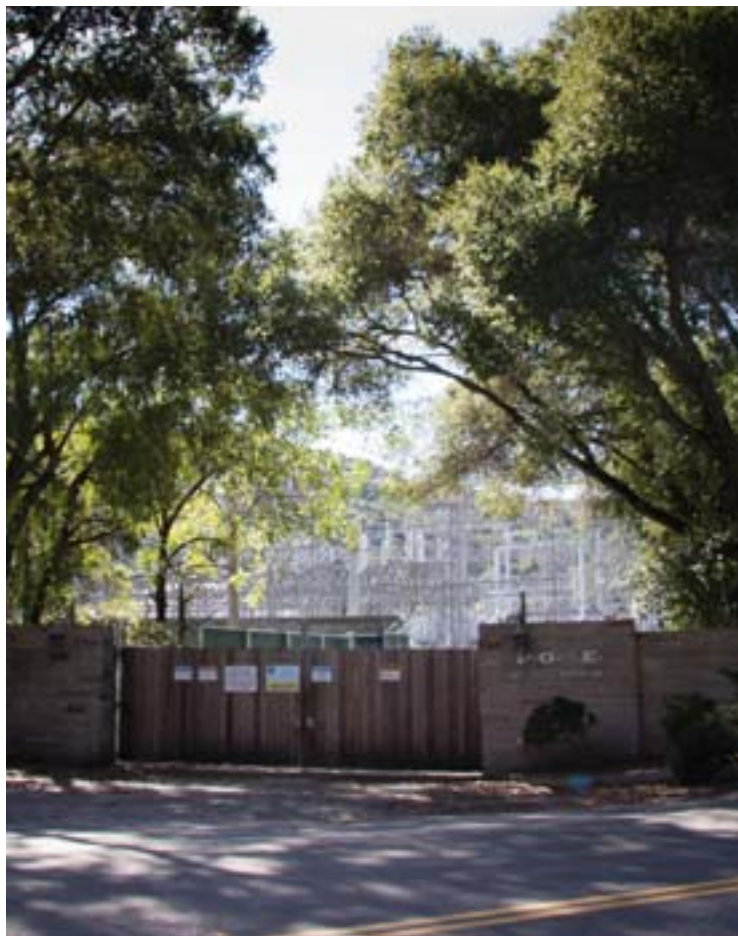
The Lost Valley PG&E substation.
