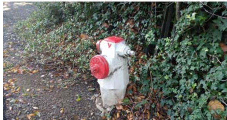
This hydrant on Charles Hill Circle in Orinda delivers substandard water flow. Photo Nick Marnell
