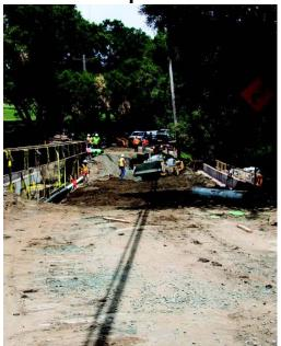
The Miner Road sinkhole repair is nearly complete. EBMUD was able to reinstall their high pressure water line within one day to put it back into service supplying water to most of Northeast Orinda. PG&E rewrapped their gas mainline for maintenance coating. The temporary steel beam support has now been removed and the sewer lines and waterline are fully operational.
