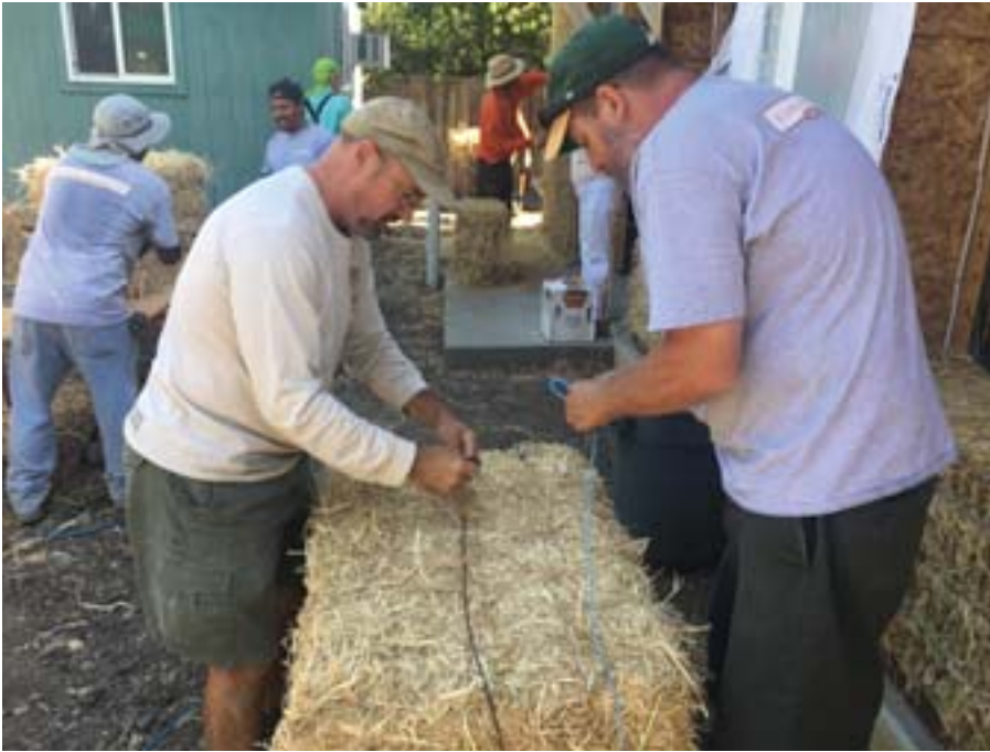
From left: Architect David Arkin and contractor Keith Kuhlmann at the straw house building site.
