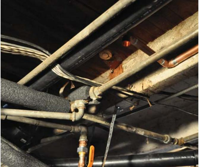
Top right, a new copper pipe is installed to replace the aged pipes.
