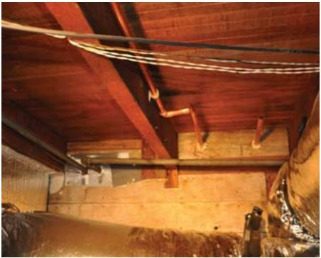
New copper piping on top and old pipes below.
