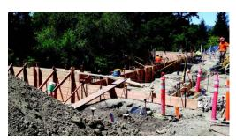
The contractor drilled and poured 36 reinforced concrete piers in May, each pier 20 feet deep and 2 feet wide. In this June photo, workers were placing reinforcing bars rebar - along the foundation. Next up comes the pouring of the slab.
