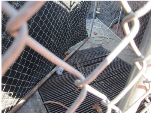
Contractor access for sinkhole inspections and repairs Photo Vera Kochan
