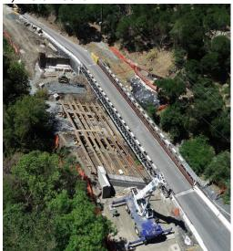
installation of "planks" spanning across the "dewatered" creek creates the false work used to build a new deck on top of it. The new roadway was moved eastward making the new bridge longer at 165 feet versus the original 100-foot long bridge.
