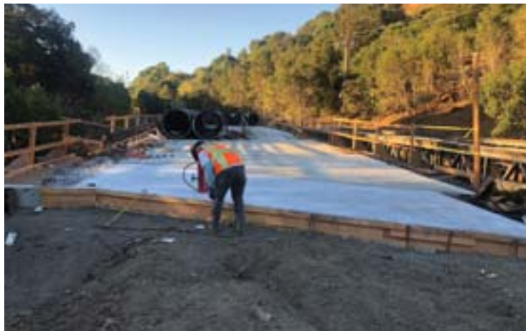
New concrete approach slab, poured Oct. 21. Photo provided
