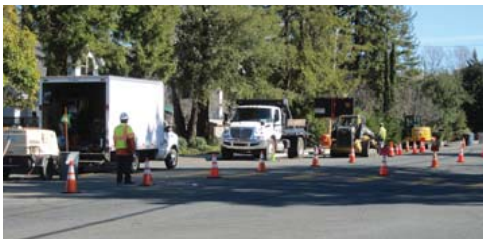
PG&E roadwork on Camino Pablo across from JMIS
