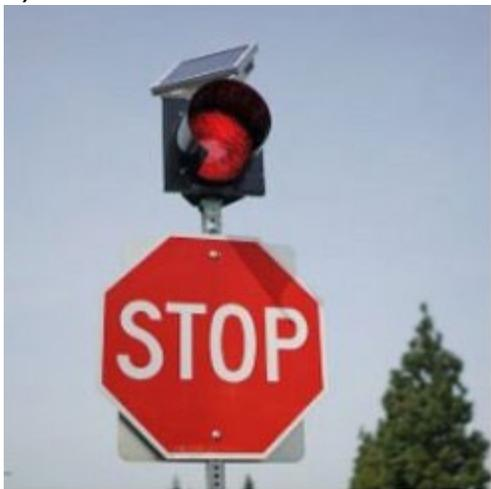
One safety countermeasure is to install flashing beacons at or in advance of intersections. Photo provided
