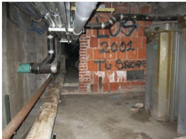
Back end of main tunnel
