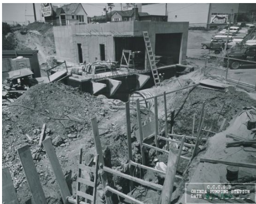
Orinda Pumping Station in 1960 Photo provided
