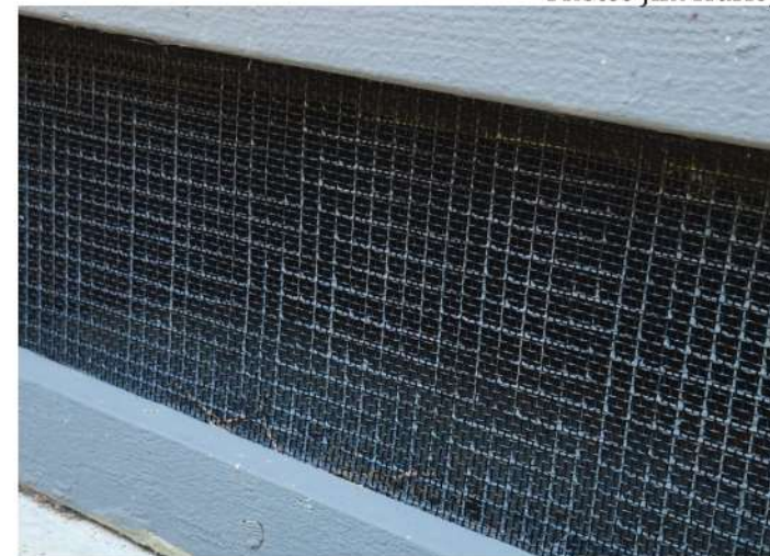
Foundation cover with additional 1/8 inch mesh
