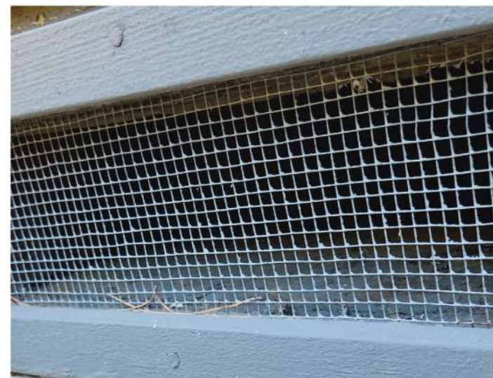
Foundation cover with 1/4 inch mesh
