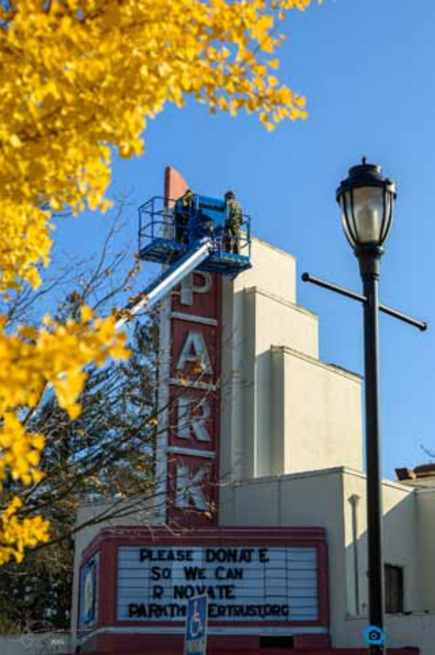
Jim Rizzo from NeonWorks in Berkeley removes the original Novial glass neon tubing from the Art Deco Park Theater tower on Dec. 5 to keep it safe and restore it.
