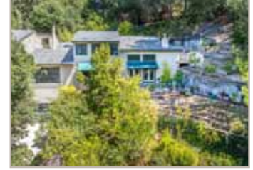
39 Mira Loma Road, Orinda
