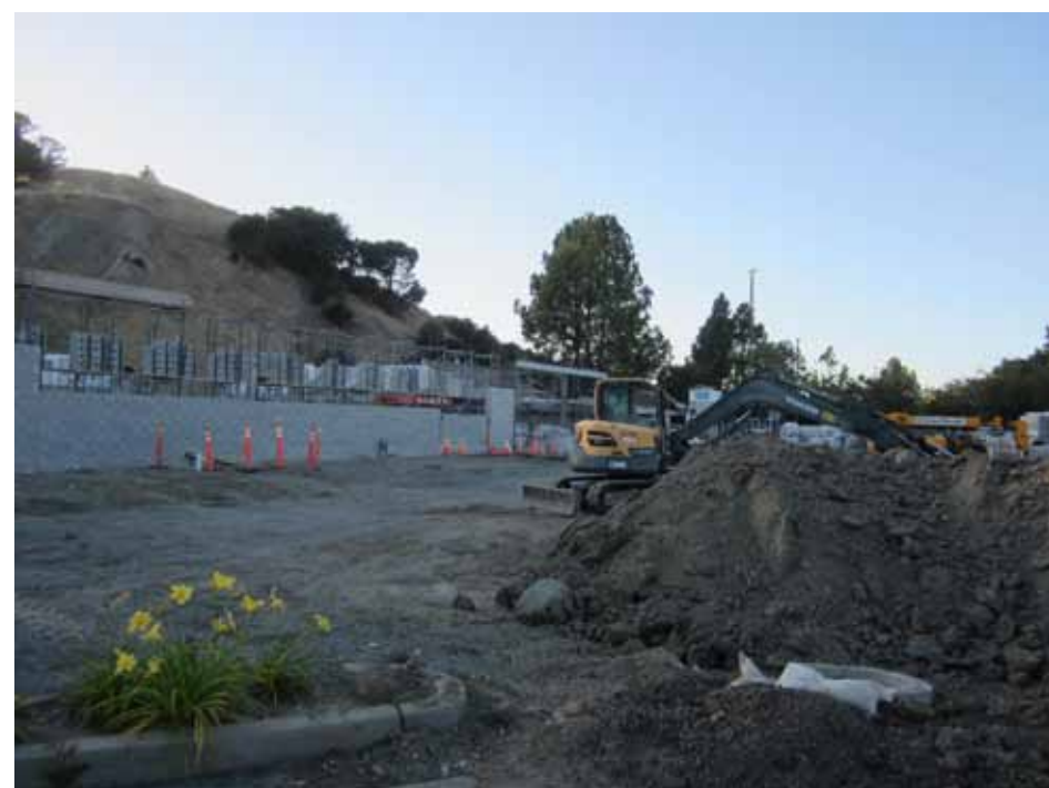
Unforeseen delays hinder Grocery Outlet construction
