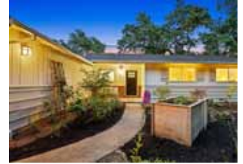
43 Monte Vista Road, Orinda
