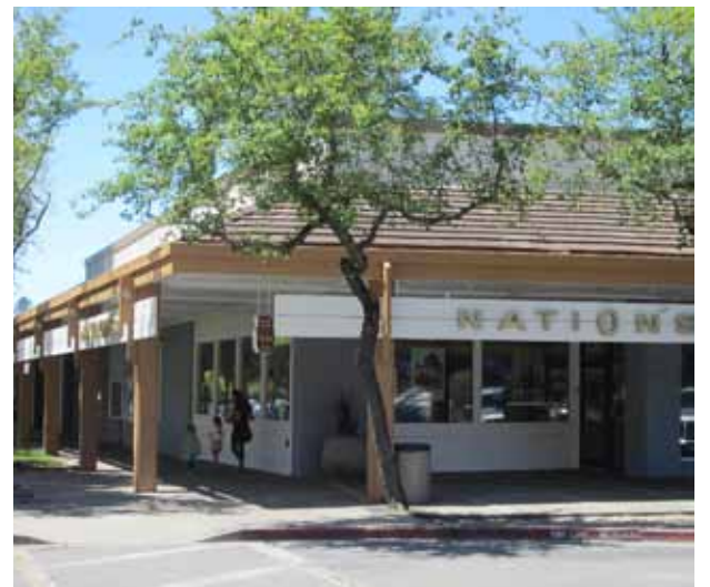
Recent cosmetic improvements at Rheem Valley Shopping Center. Photo Vera Kochan
