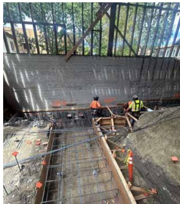
Foundation work at the Park Theater in progress. Photo provided
