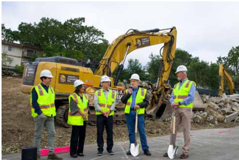
Lafayette mayor Carl Anduri speaks at the June 25 ground breaking of Oak Hill, an 85-residence luxury condominium community at 1001 Oak Hill Road.
