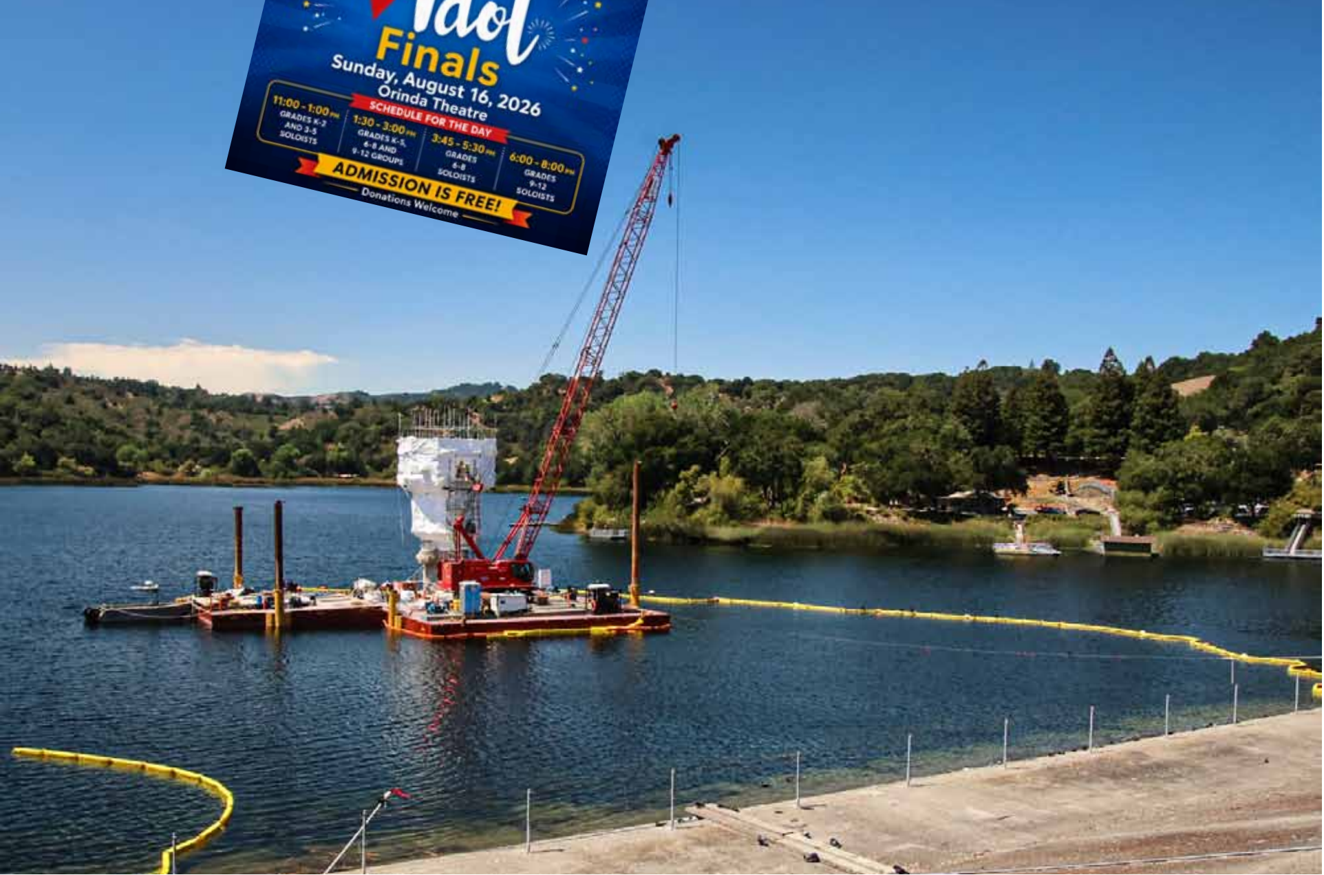
Retrofit work on Lafayette Reservoir tower. Photo Sora O'Doherty
