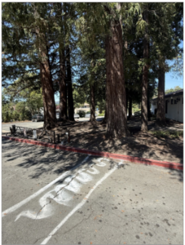
Moraga Library redwood trees pose an unacceptable risk to foundations and utilities.
